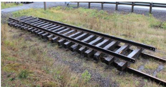
Left: Panel track for Chapel Road crossing ready to be install the next weekend
