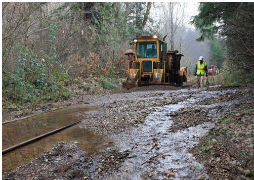
Left: The Ballast Regulator clearing the small slide near mile post 2.5
